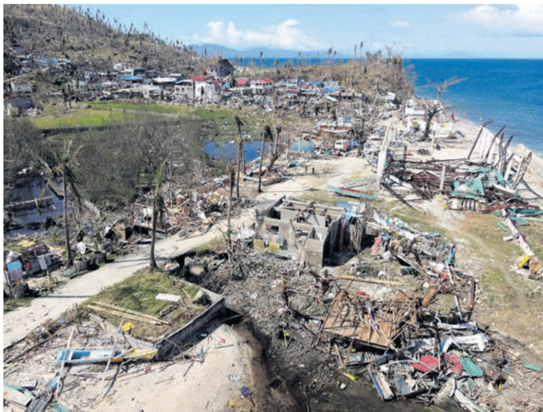
In this photo provided by Greenpeace, damaged homes due to Typhoon Rai lie along a coastal village in Surigao City, southern Philippines Monday Dec. 20, 2021.
